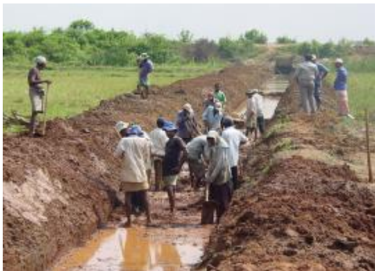
Community members participate in building an irrigation channel
